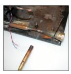
**9.** Bend the filter-drier up and out, away from the mounting base. Clean the condenser discharge tube near where it joins to the filter-drier with the abrasive cleaning pad (079-2010).
