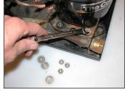
from the old compressor base and dispose of the compressor according to EPA regulations.
