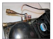
6. Remove the fasteners holding the compressor to the condensing unit mounting base as shown in the photo to the right. Retain these fasteners for use in a later step. Remove the
