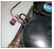
5. Use the tubing cutter to cut off the suction line as close as possible to the compressor suction tubing stub. It is not necessary to de-burr the end of the cut tubing, as this section will be discarded and replaced with a new piece. Heat the end of the suction line quick connect fitting with a torch and remove the short section of 1/4" tubing from it. Do not overheat the body of the quick connect fitting.
